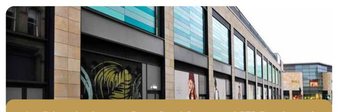
A collaboration between Paroc Panel System and BTS Facades and Fabrications, the Vantage® PPS system is made up of industry leading, Euroclass A2-s1-d0 rated sandwich panel with a structural (Euroclass A1) stone wool core, combined with the Vantage® SF rainscreen front face, tested to the latest BS8414-2:2020 standard.
